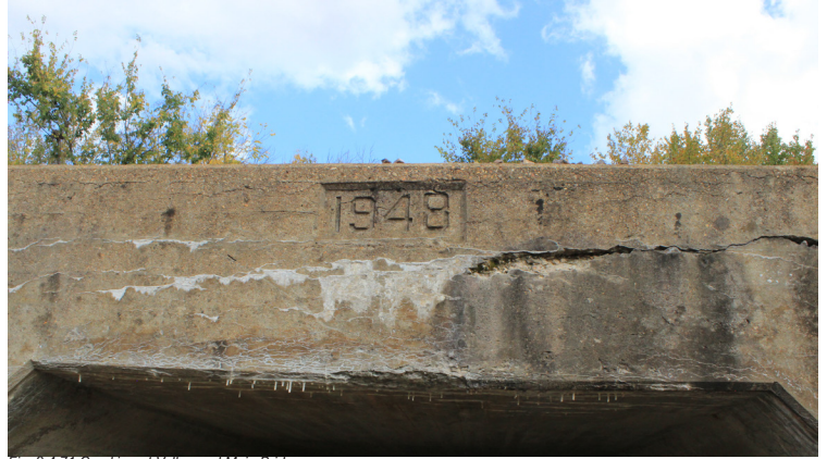
Fig. 2.4.71 Cracking at Valley and Main Bridge
