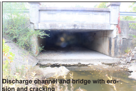
Concrete was poured to stabilize bridge foundation
