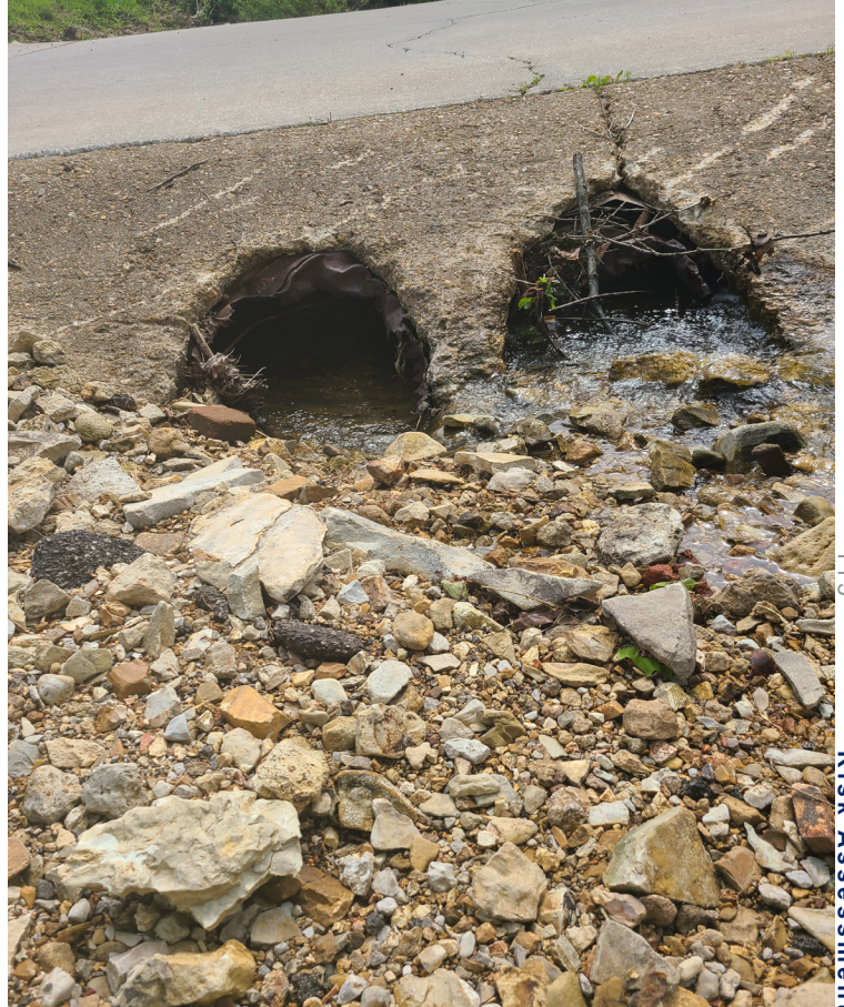
Fig. 2.4.74 Erosion at Storm Drains and Debris Carried
