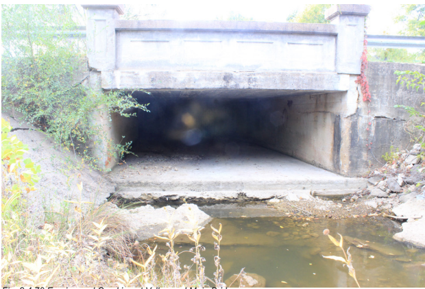
Fig. 2.4.70 Erosion and Cracking at Valley and Main Bridge
